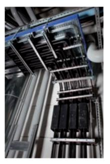
Our bus ducts are suitable for power distribution feeding and branching and are designed according to customers' specific needs. The modular design of the bus ducts means that they are well suited for a variety of special applications in both new installations and modernisations.
